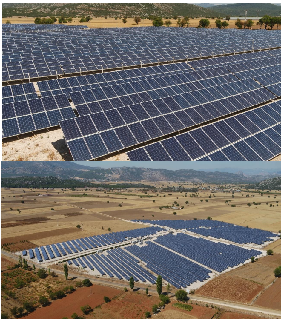
Figure 14: View of the Photovoltaic Solar Power Plant installation
